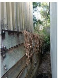
Some retaining wall timbers require repair / reinforcement / replacement.
