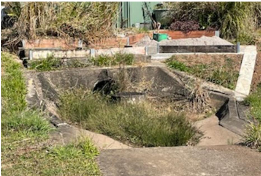
Fig 1 - Outlet structure of Upstream Basin
